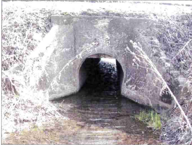
Figure 4 Upstream (north) end of railroad culvert
