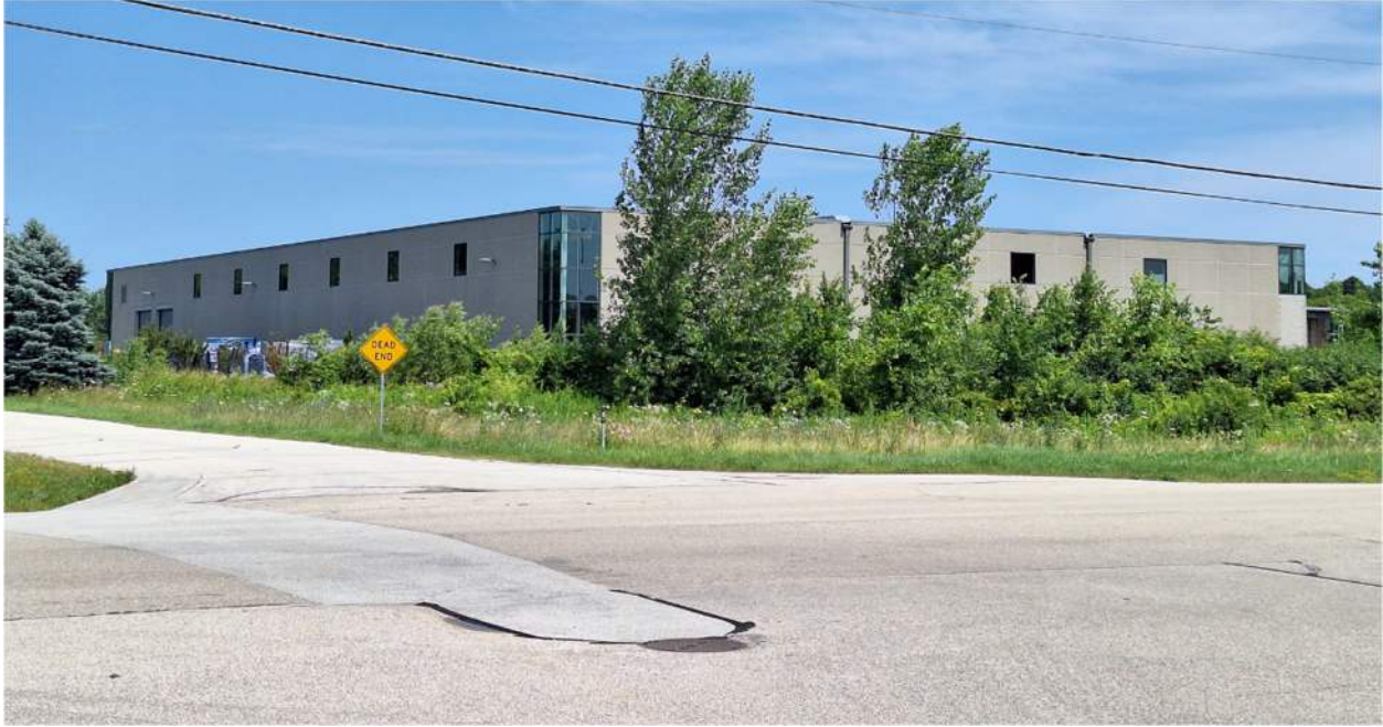
Exhibit E (KD Glass Loading Dock & Storage from N46W22992 Charlotte Way)
