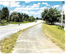
Transition from a rural roadway to an urban roadway section to minimize right-of-way impacts.
