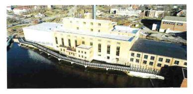
systems. Substantial vertical grade difference is present throughout the corridor as the path traverses along the Rock River on land, and then transitions to the ten-span bridge system which is set to match future doorway connections on the repurposed Powerhouse building. The path is designed to accommodate both the horizontal and vertical locations of the various floors of the old building. Batterman provided all project services (except for structure design) for this TAP project.
