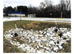
Drainage design was key in areas where the path was close to the roadway.
